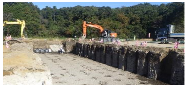
Photo-2 Excavation of improved constructed by GeoPilot-AutoPile
