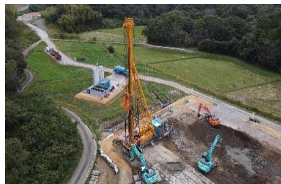
Photo-1 Construction status
