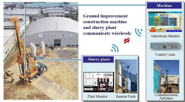
Figure-1 GeoPilot-AutoPile Systems Configuration Overview
