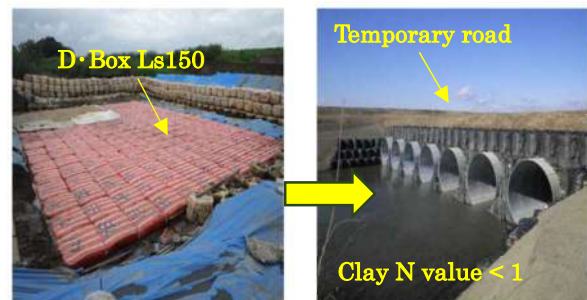
Photo-4: Temporary bridge foundation in Ramsar Convention wetlands
