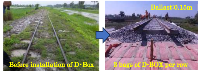
Photo-10: Improvement of the railway subgrade using D·Box
