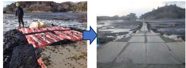
Photo-9: Construction road on the pond of designated National Park Area
