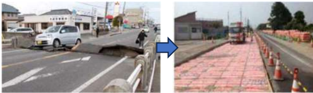
Photo-6: Liquefaction Mitigation Measures
